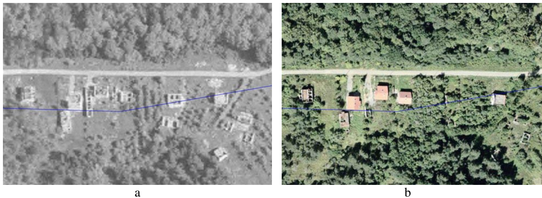
Figure 2. The demolished houses from 1999 – 2001(a) were reconstructed in 2006 (b) [Bajic, Krtalic 2009].
